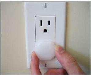
A safer solution is installing tamper-resistant outlets. These specialized outlets have been so effective in preventing injuries to children that the 2008 National Electrical Code requires that tamper resistant outlets be installed in all new homes constructed," says ESFI.
